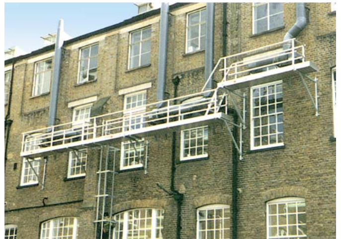
Wall bracket mounted access to soil pipes above busy thoroughfare - City College, London.
