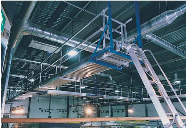
The permanent installation of a suspended Spandeck walkway in the Royal Signals Museum provides access to roof work areas such as air conditioning without closing exhibition to the public.
